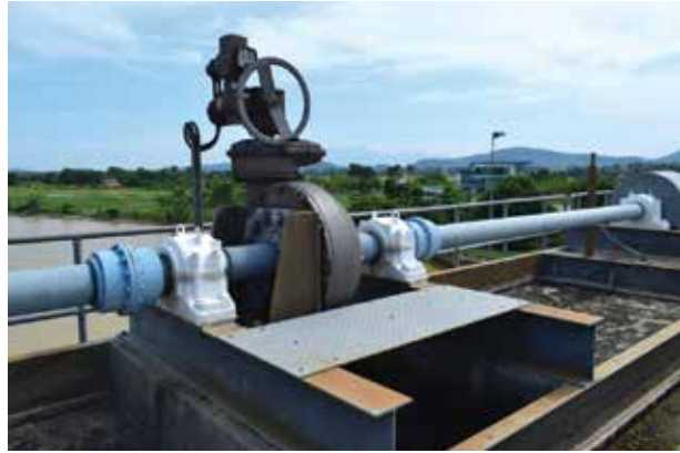
Figure 3: The Actuator can be operated in manual operation
